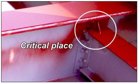
Fig. 2: Critical fatigue construction detail of the bridge
